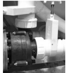
Slice Valve and Pump Union
