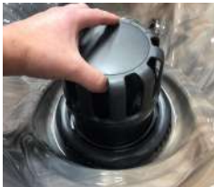
Pull Up to Remove Floater Assembly
