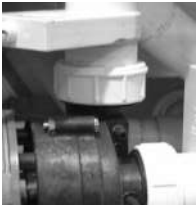
Slice Valve and Pump Union
